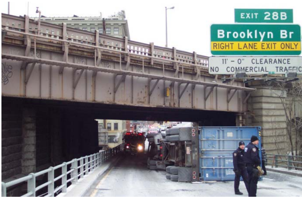
Figure 4: Low-clearance underpass in New York City (Yanev, reproduced in Latour 2004).
